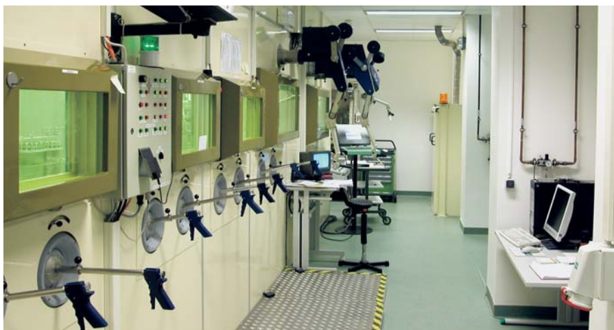
Hot cells for investigating irradiated reactor material.
