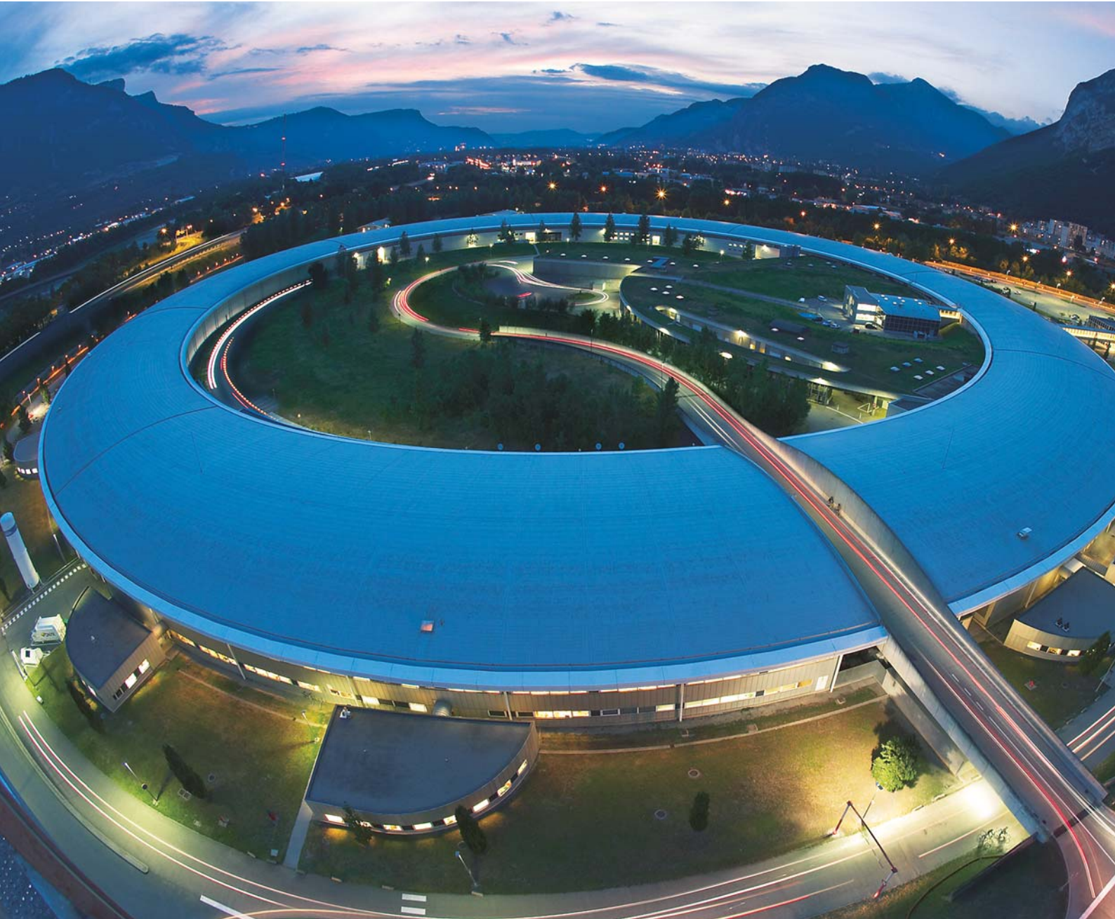
European Synchrotron Radiation Facility.
