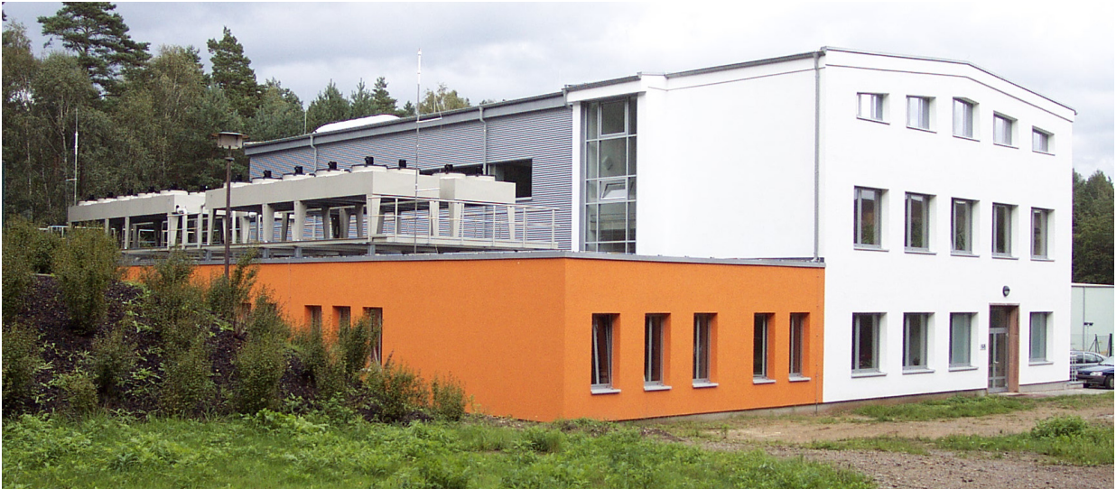
Fig. 2.3 TOPFLOW building with dry cooling system on top of the roof of the left wing
