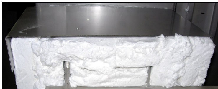
Fig. 2.11 Thermal insulation with Multitherm and covering with stainless steel sheets
