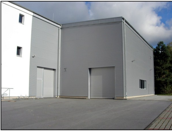
Fig. 2.2 New wing of the TOPFLOW building
