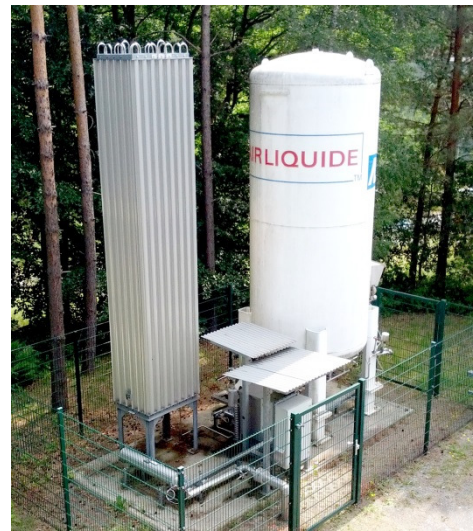
Figure 2.3: Nitrogen supply unit
